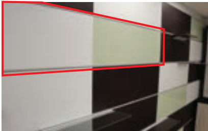
Snap in panels installed
